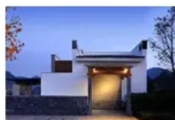
Household Energy Storage
