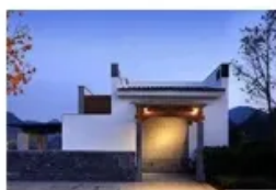
Household Energy Storage
