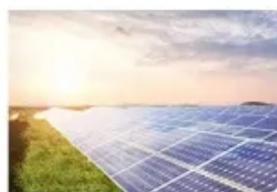
Energy Storage System
