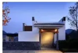
Household Energy Storage
